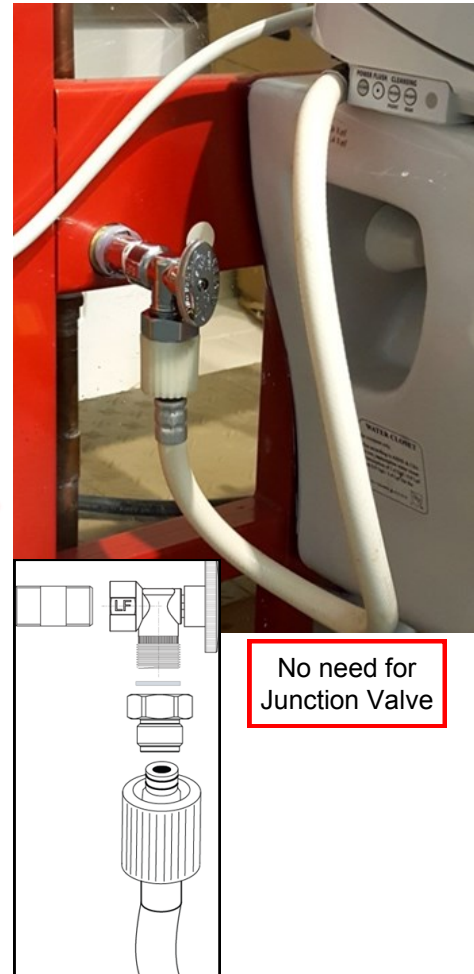
Replacement Installation Set-Up
